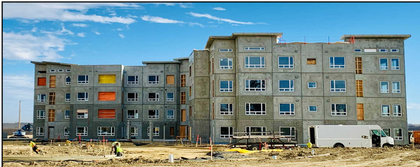
Photo taken on October 25, 2019. Front view of Chinook Villa, with top roof panels up and most of the windows in. The curbs and roads are under construction for the duplexes to be built in early spring. A newly added option is to lease a duplex with an unfinished basement for a savings of approximately $40,000.
